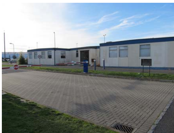
Figure 23 Portacabin Offices currently occupying Site 5
