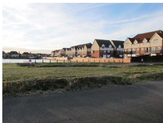
Figure 32 Site 8 looking towards Hobart Quay
