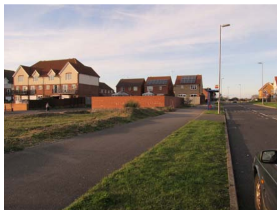
Figure 31 Pumping Station on Site 8
